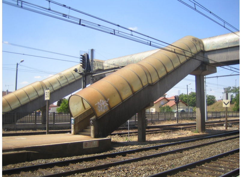
Figure 52 : Passerelle gare de St Priest
